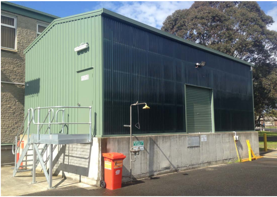
Figure 13: Traralgon Water Treatment Plant - Chemical storage facility Traralgon Water Treatment Plant upgrade to chemical storage facility and bund.
