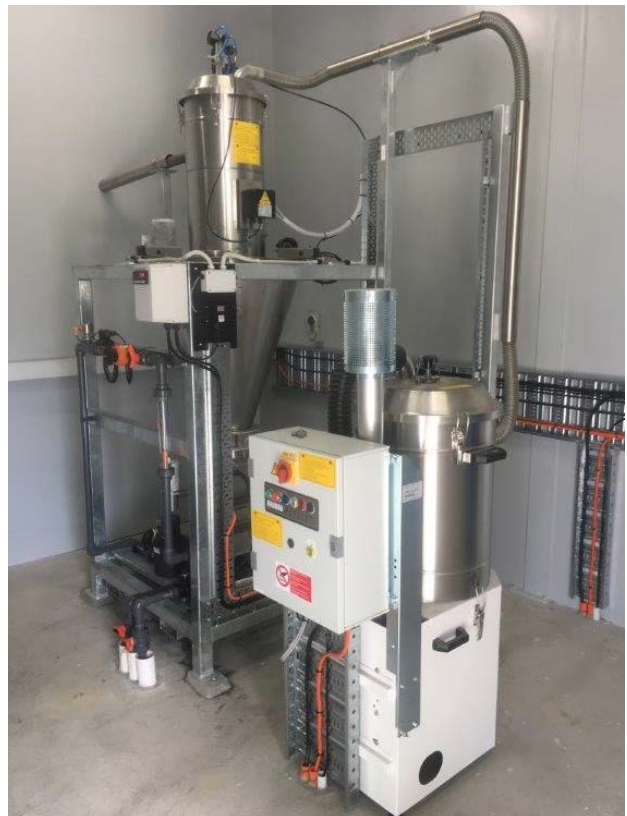
Figure 8: Heyfield water supply locality project – Activated carbon system Heyfield Water Treatment Plant upgrade to powder activated carbon system for water quality taste and odour water quality aesthetics management.
