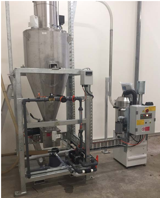
Figure 7: Maffra water supply locality project – Activated carbon system Water treatment plant upgrade to powder activated carbon system for water quality taste and odour water quality aesthetics management.
