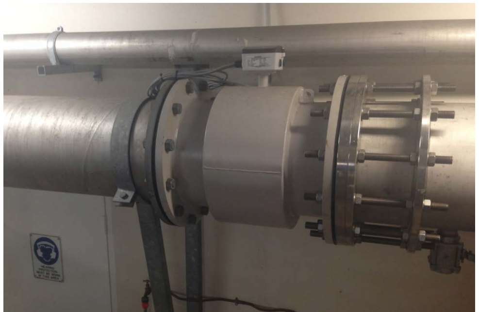
Figure 14: Traralgon Water Treatment Plant – Outlet flow meter
