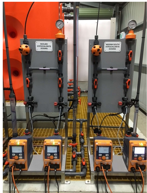
Figure 7: Neerim South water supply locality project – Disinfection system upgrade
