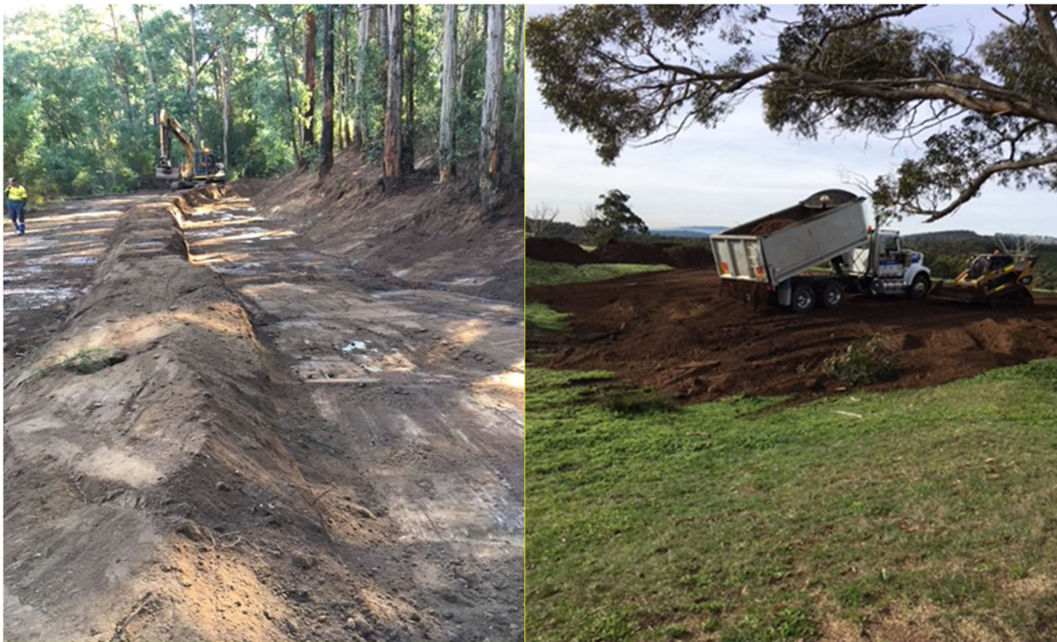
Figure 15: Mirboo North Weir – Desilt clean-up activities
