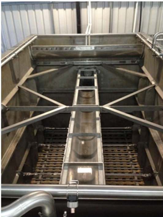
Figure 13: Traralgon Water Treatment Plant – Filter Upgrade
