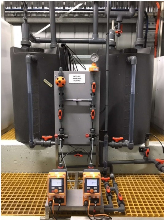
Figure 7: Neerim South water supply locality project – Disinfection system upgrade
