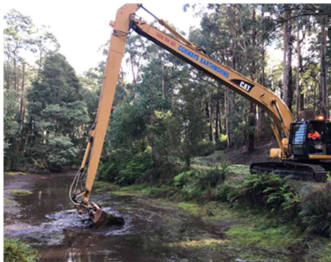
Figure 16: Mirboo North Weir – Desilt clean-up activities
