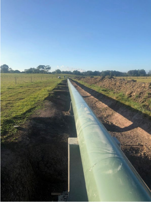
Figure 8: Traralgon raw water main upgrade
