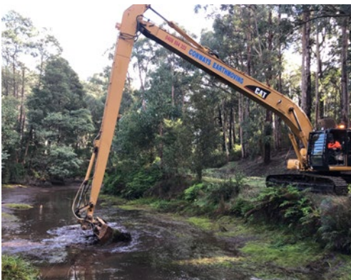
Figure 16: Mirboo North Weir – Desilt clean-up activities
