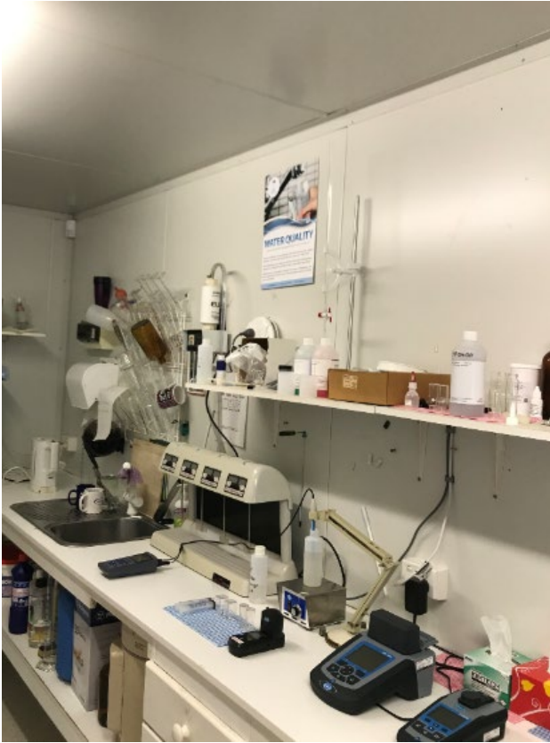
Figure 15: Refitting of Neerim South WTP laboratory
