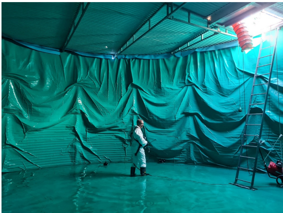
Figure 12: Cleaning and disinfection of drinking water storage tank in Noojee
