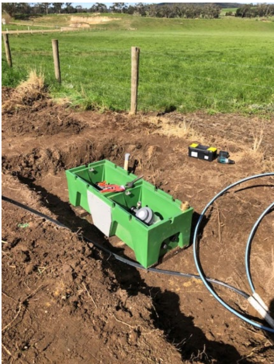
Figures 14: Installation of automatic flushing devices for managing water quality at extremities of system
