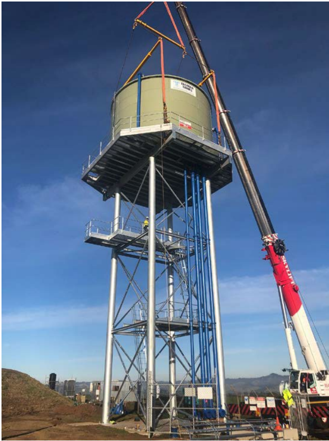
Figure 13: Replacement of water storage tank assets, Warragul South
