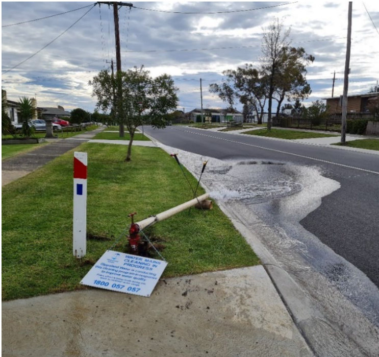
Figures 8: Preventative Air Scouring mains cleaning in Trafalgar and Morwell
