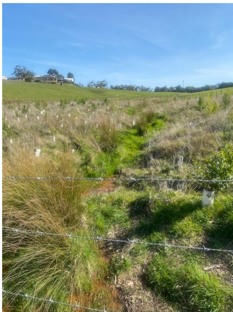
Figure 9: Revegetation at Willow Grove stormwater for water quality improvement
