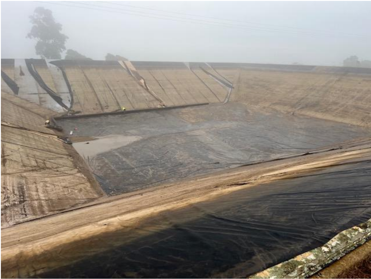
Figure 19: Warragul WTP Basin cover and liner replacement project
