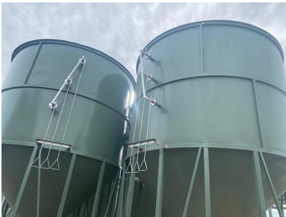
Figure 13: Installation of new sludge silos at Heyfield WTP
