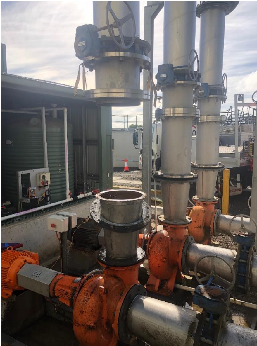
Figure 17: Replacement of non-return valves on pumps at Moe WTP
