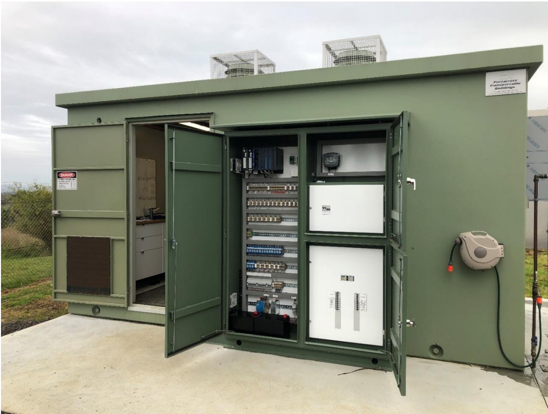
Figure 14: Installation of a new secondary disinfection site at Rosedale
