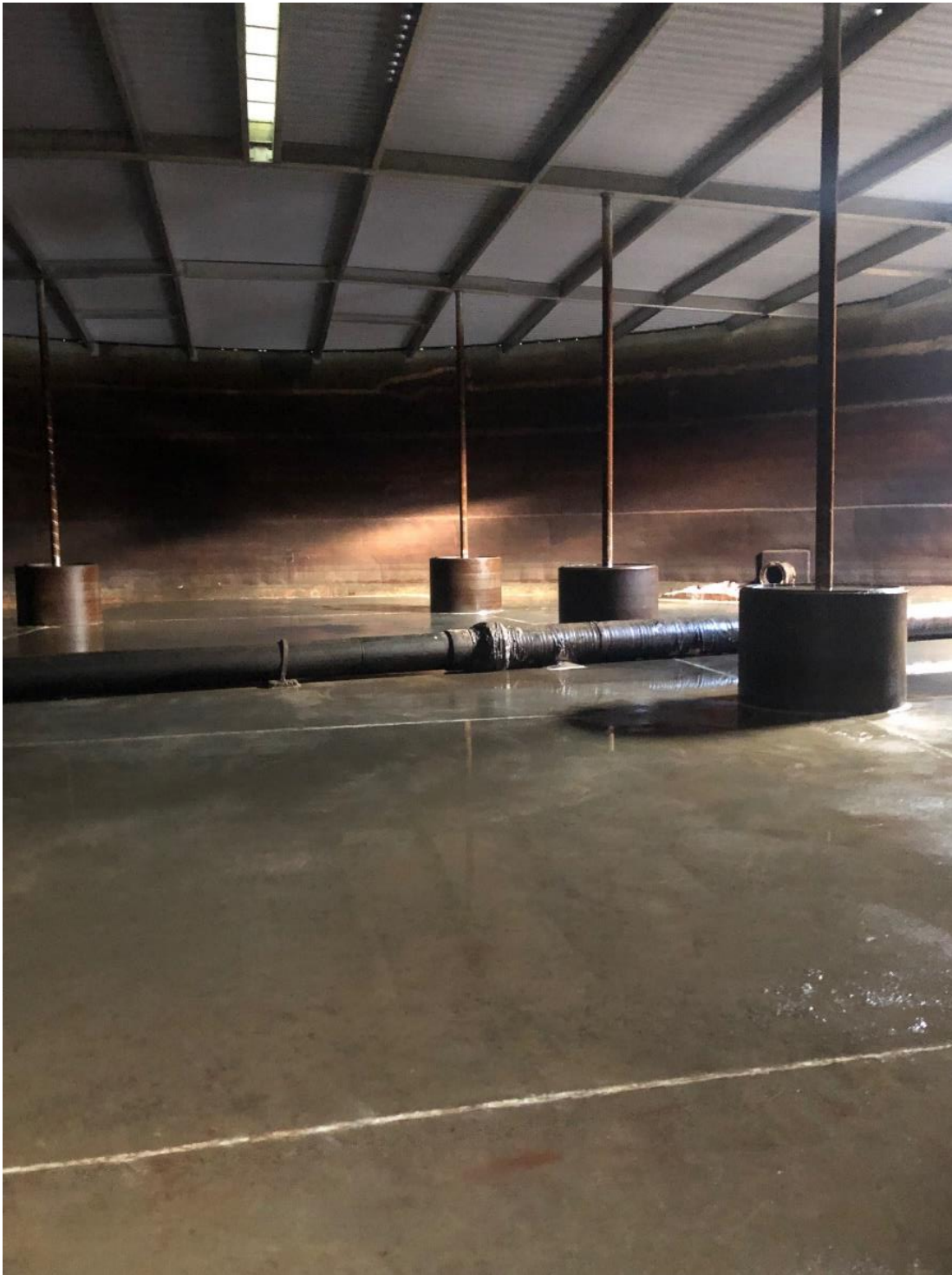
Figures 16: Cleaning the inside of the contact tank and Warragul WTP
