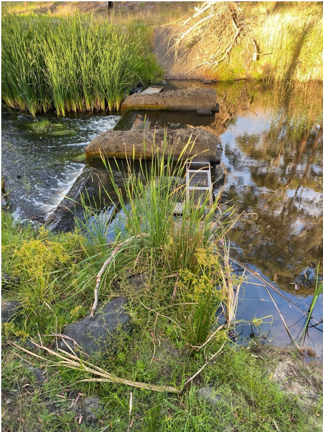
Figure 18: Undertaking maintenance on the Merriman Creek weir at Seaspray
