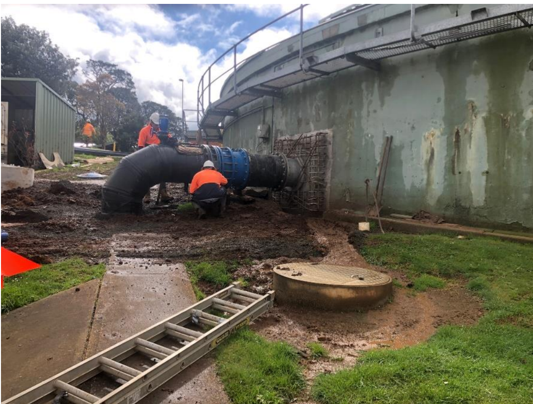
Figure 15: Installation of new pipework into the Contact Tank at Warragul WTP
