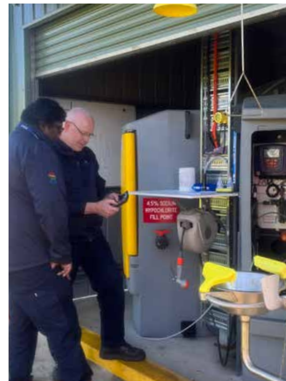
Figure 11: installation of a new secondary disinfection site at newborough
